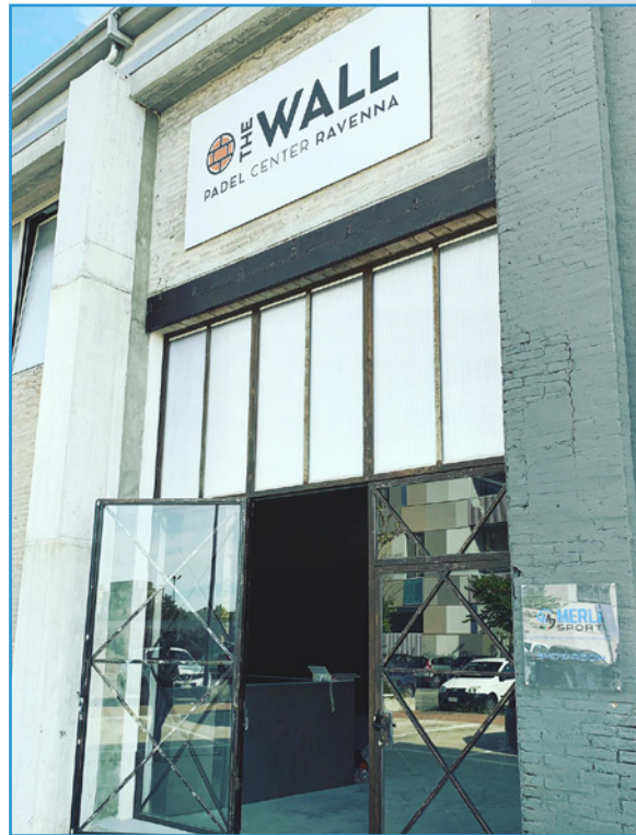
SHOWROOM RAVENNA / ESTERNO
